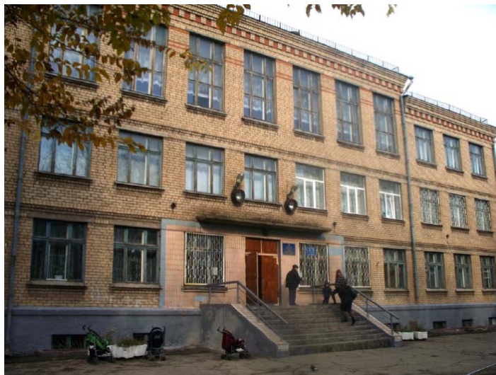
Fig. 1. The 3-storey school building constructed in 1960
